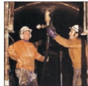
Grout injection and backfilling
